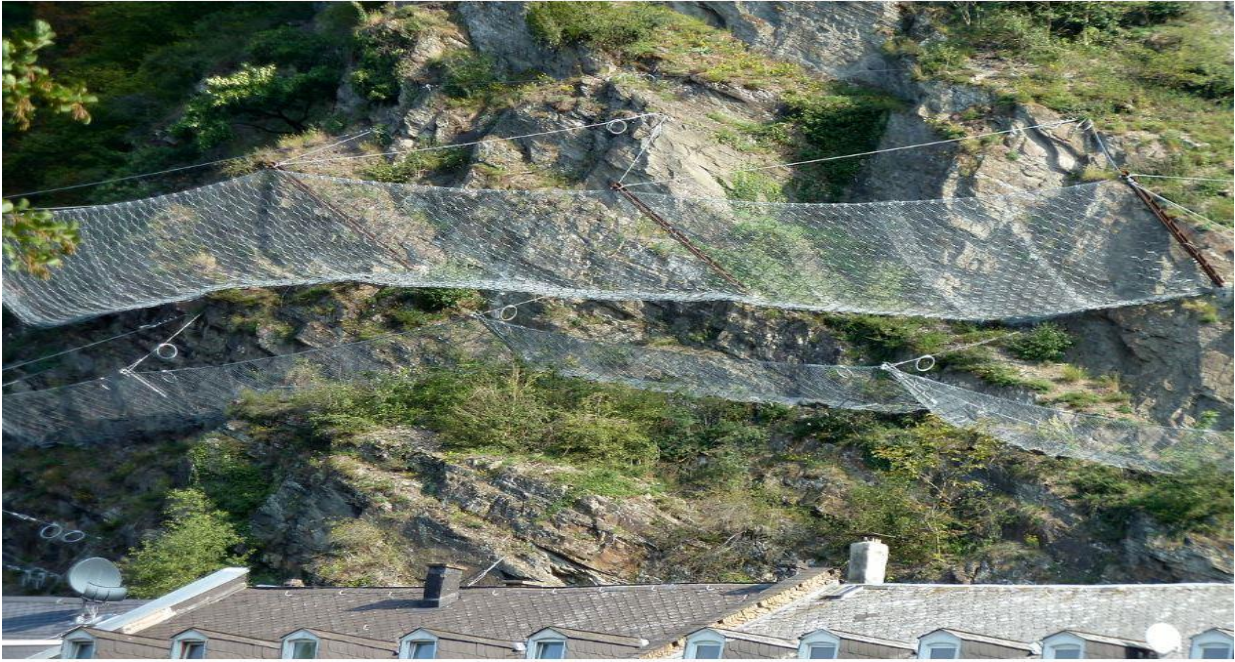
Figure 13: Rockfall Barrier.
