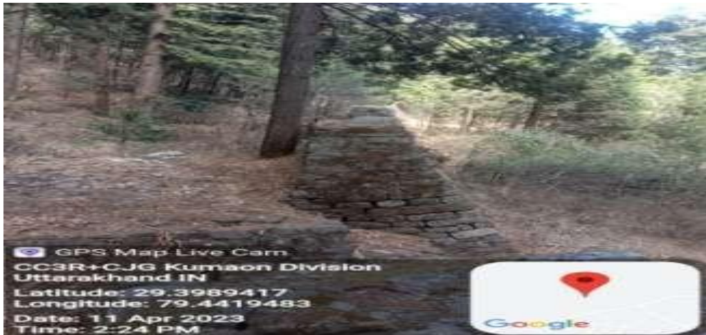
Figure 6: Retaining Wall structure above the Kilbury Road
