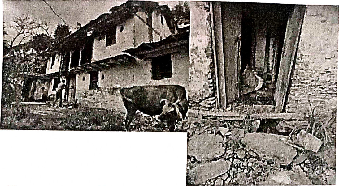
Figure -3 A house with water seeping out from beneath its floor.
