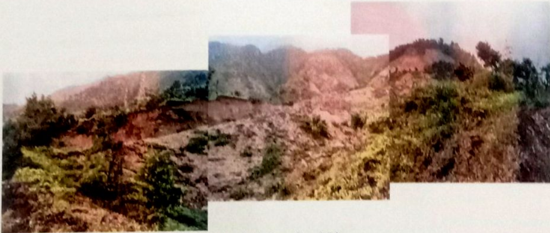
Longitudinal View of Landslide
