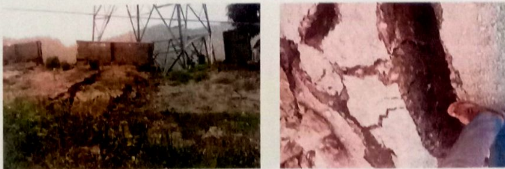
Longitudinal cracks on Ground
